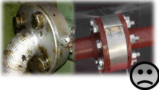
Held tight against the flange, generally with poor connection design with open gaps.
