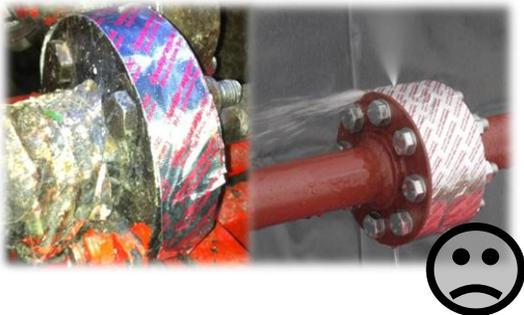
Convenient tape solution, should be wrapped with 50% overlap, all the way down to pipe.
